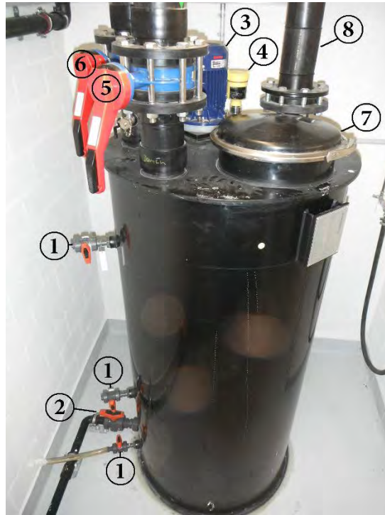
Figure 5.2. Urine storage tank, at the basement of EAWAG office building. 1) Sample ports. 2) Effluent port. 3) Mixer. 4) Level sensor. 5) Women's toilet influent. 6) Men's toilet influent. 7) Hermetic tight. 8) Ventilation.
