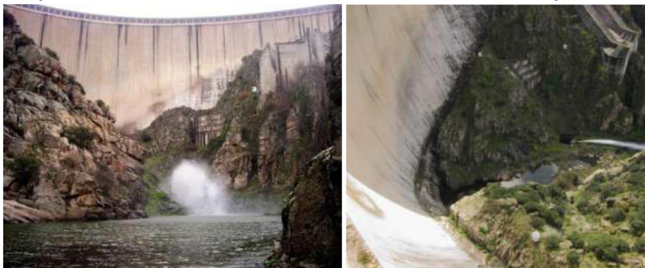
Fig. 5.4. Almendra dam shot from downstream (left) and upper view (right). The plume is the ‘ecological flow’ released through a Howell valve that never surpasses 500 liters per second. The water table in the forefront is contained in a little shock-absorber reservoir. Pictures taken by Ignacio Rodríguez.
